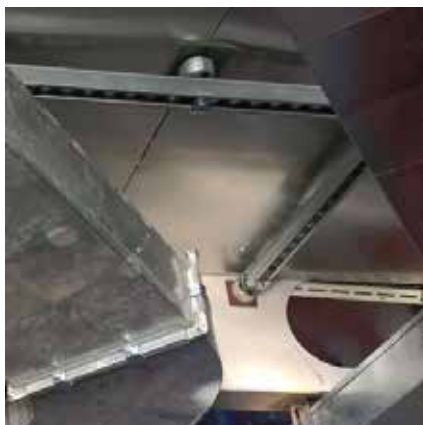
Vibration-isolated ceiling suspension
